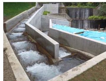
e) Proposed fishway installed in check dam (10m height)
